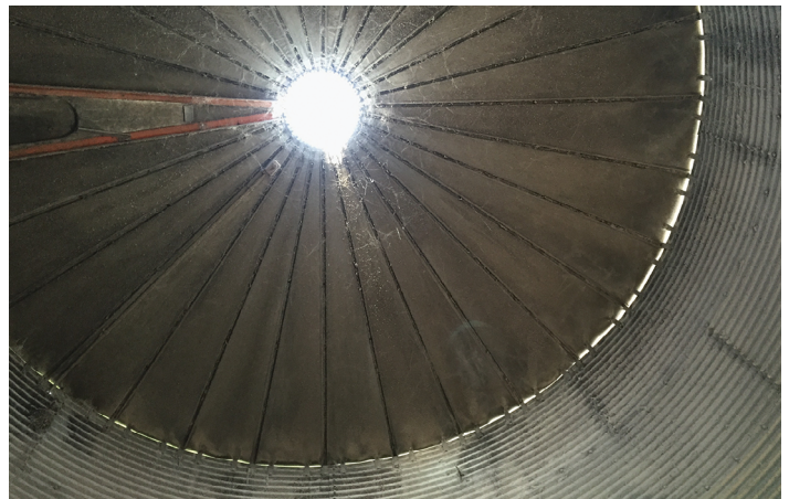
Figure 5. Interior of a grain bin.
